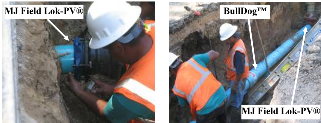
Figure 11: Joint Restraints at Tie-In A
